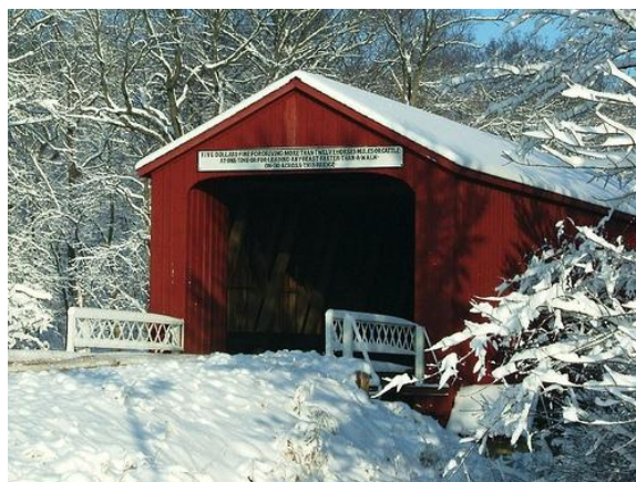
Figure 60: Red Covered Bridge
