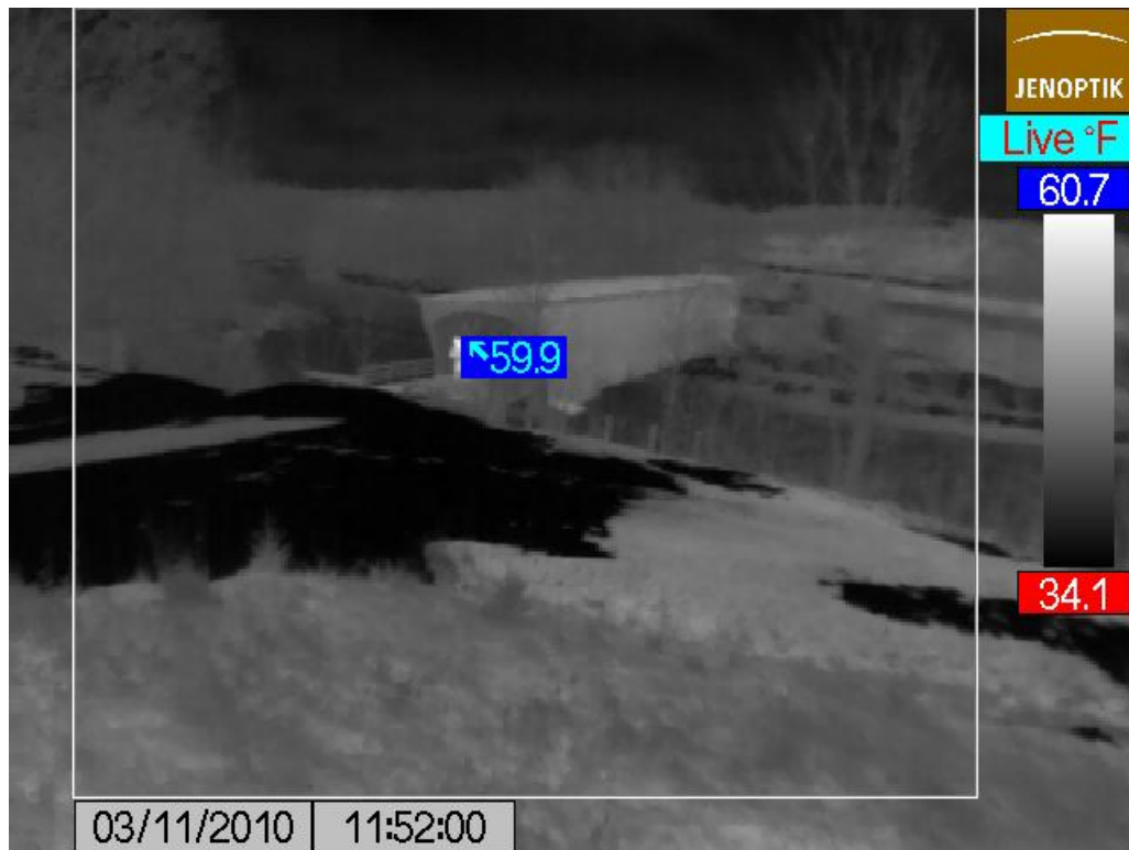
Figure 23: Infrared Camera Image at Holliwell Bridge
