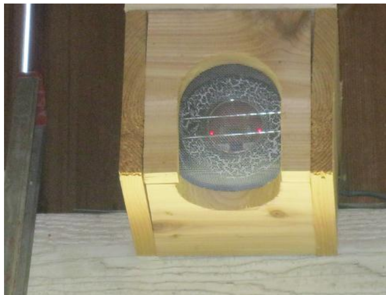
Figure 31: Cutler-Donahoe Flame Detector that is set off
