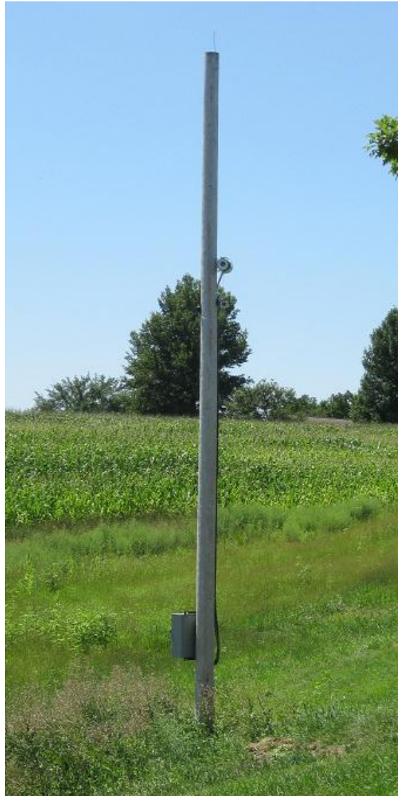
Figure 65: Complete Pole after Installation
